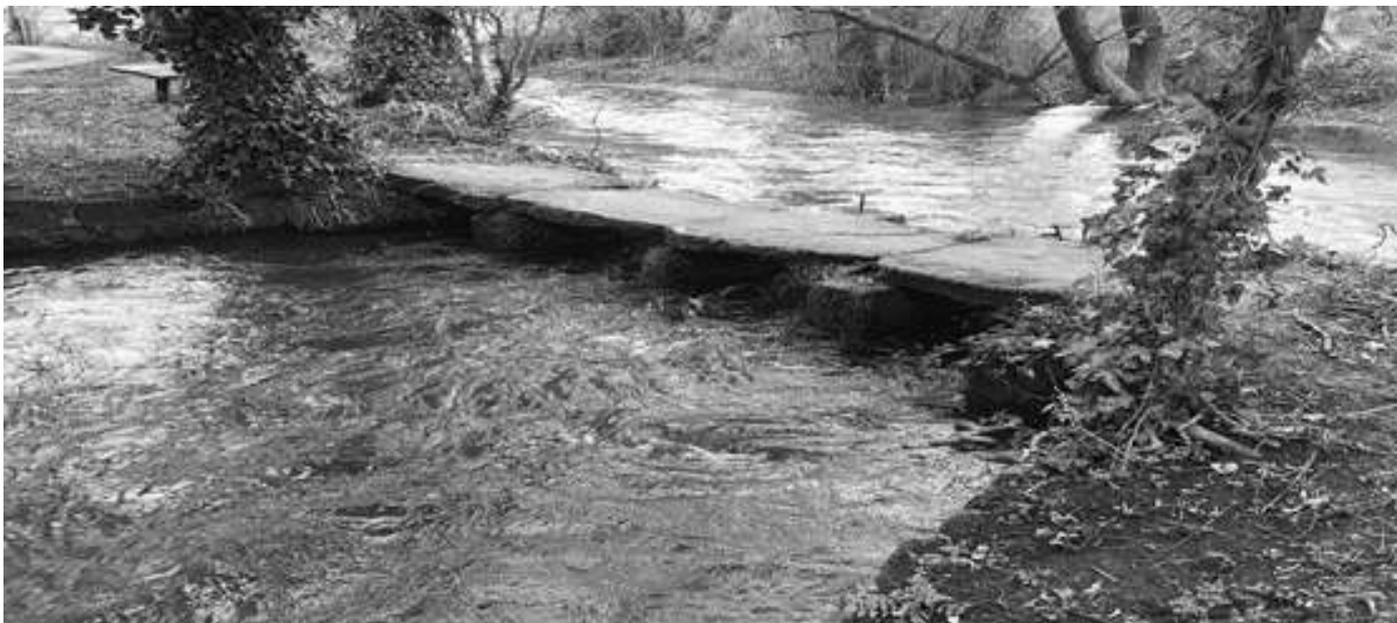
*“Clapper bridge, probably seventeenth or eighteenth century, consisting of three large limestone slabs supported on four low rectangular piers, with projections to west with grooves for hatches. A good unaltered example of this type of bridge”.*
