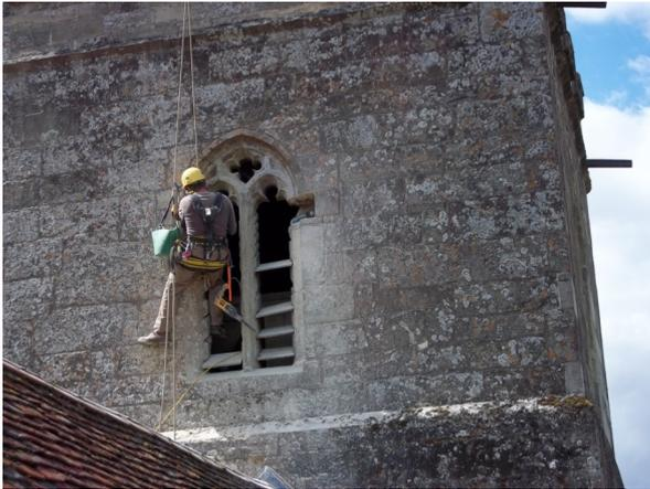
By securing their ropes on the top of the tower, and using special karabiners, they are able to descend to the appropriate spot and stop. They then have both hands free to work while hanging in a seat from the rope. When finished, they use the karabiner to ascend to the start point.
